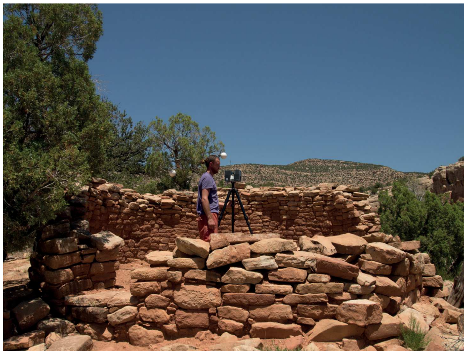
Figure 7. Laser scanning of the Site 5MT13446, the tower that is located approximately 120 m SE of the Sunny Alcove site. Photo by J. Nawrot.
